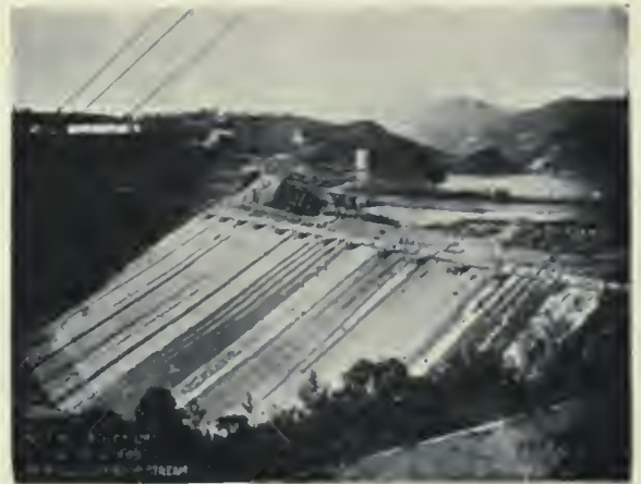
Necaxa dam, lower rockfilled toe with masonry face.
